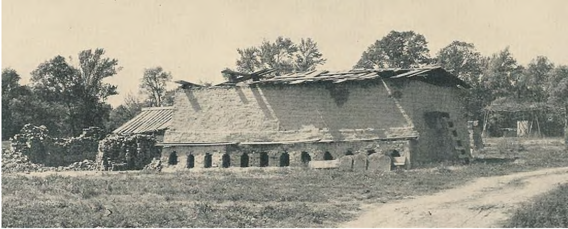
Figure 7. The kiln used to fire the bricks for the memorial house.
