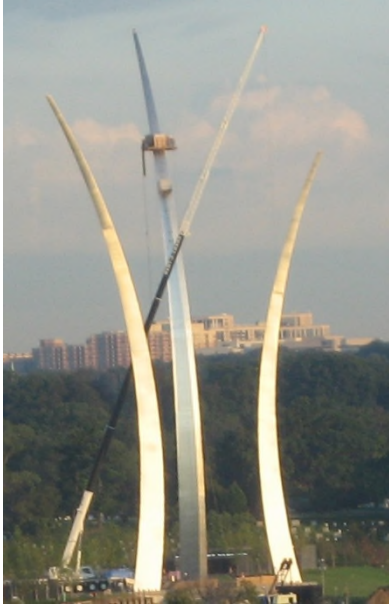
Figure 2. The New Air Force Memorial, still under construction.
